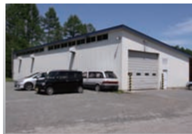
⑧端野剥き玉加工施設
